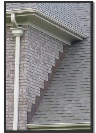
**12. Flashing:** All flashing must be copper or painted galvanized metal. Exposed galvanized or aluminum flashing is not permitted.
